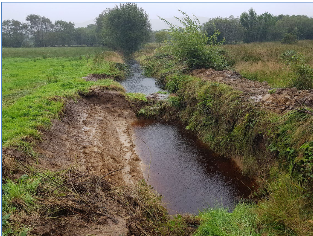
Figure 11 In-ditch wetland under construction. Note reprofiled drain with shelves of different depths creating different depths and widening the drain. Earth bunds are also visible as barrier to slow the flow of water within the drain. (source: Pearl Mussel Project)
